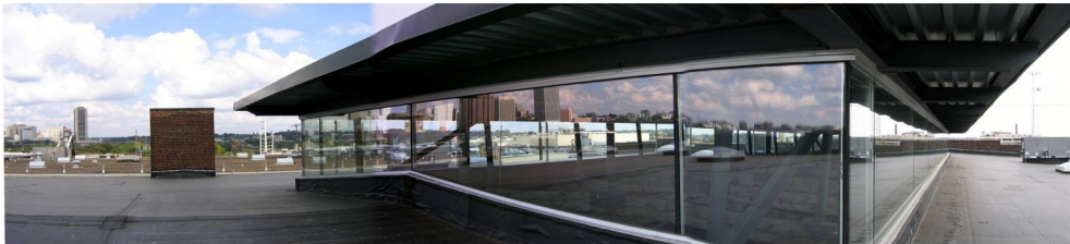
PHOTO / EXTERIOR VIEW OF ROOF MONITOR
