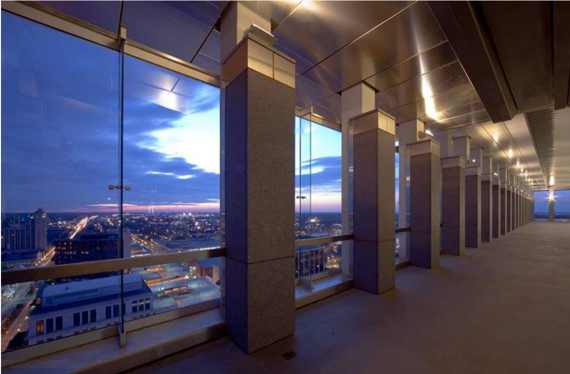
Detail of renovated skydeck
