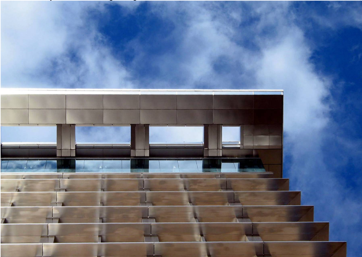
Front elevation / roof detail
