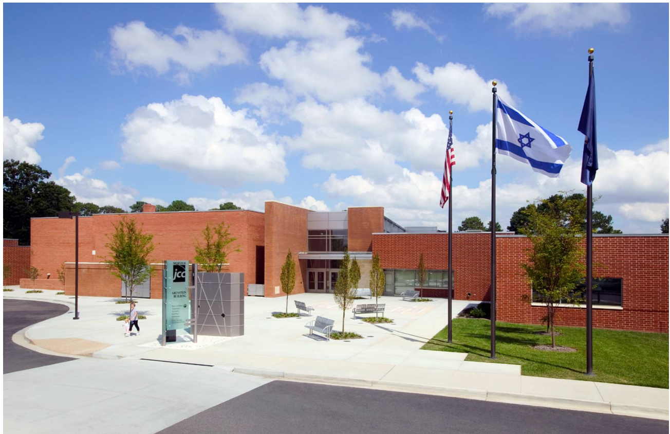
View of new addition from main parking lot
